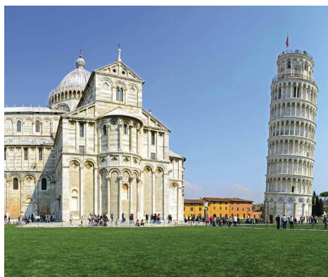
Leaning Tower of Pisa
